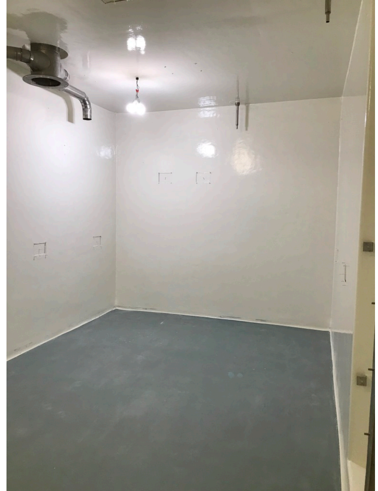
2 nd layer of 2 part epoxy (sand and fully clean between applications)
