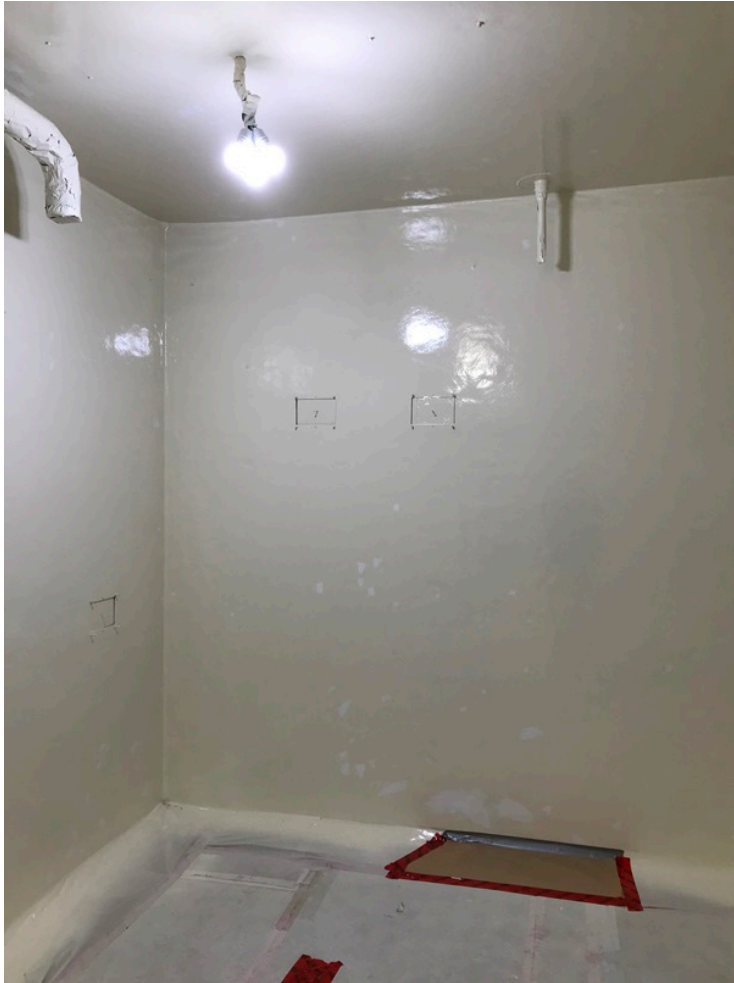
1 st layer of 2 part epoxy
