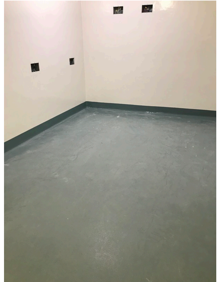
Reinstallation of covered baseboard assembly
