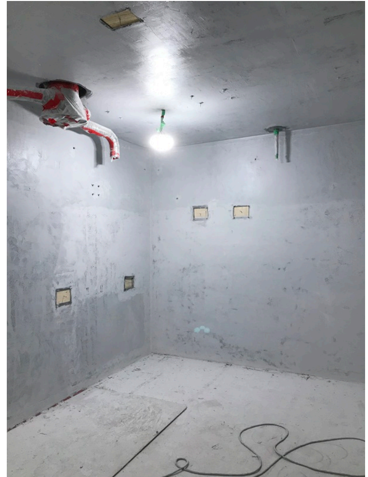
2 nd later of filler (grind between each layer with grinders)
