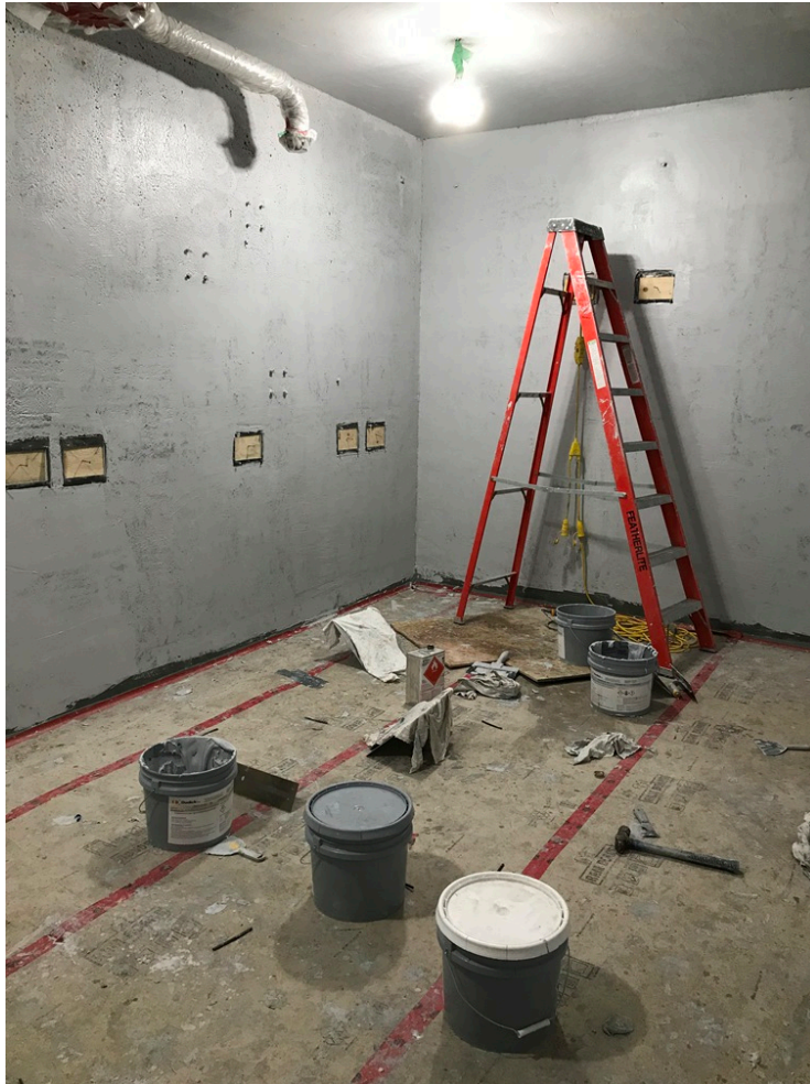
Sealant and 1 st layer of filler
